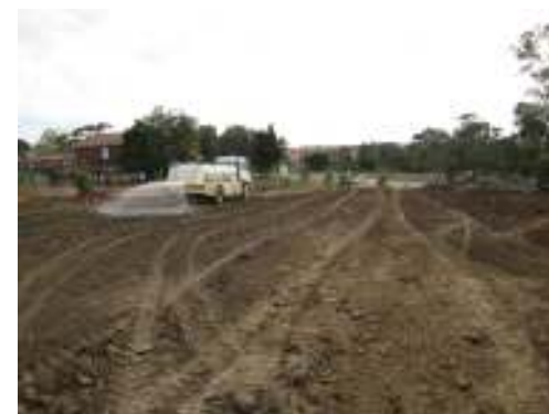
Moisture conditioning of the fill
