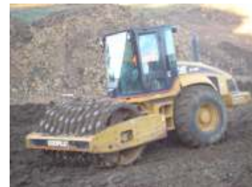
The compaction process
